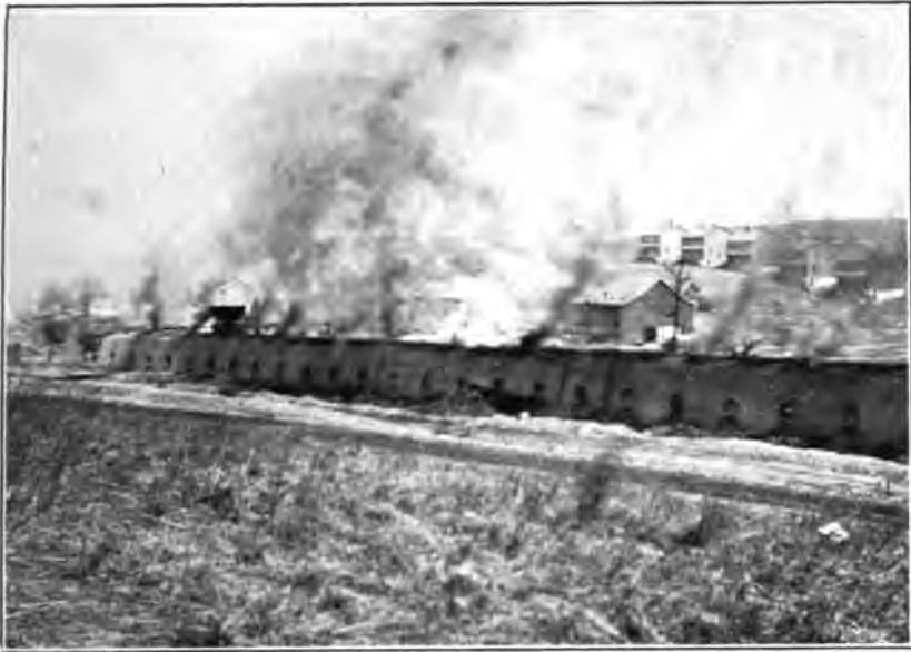
COKE OVENS IN CONNELLSVILLE REGION A way station for fuel en route from coal pit to blast furnace
